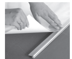
Step C: Firm pressure onto surface
